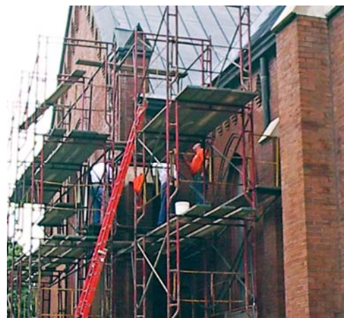
Crew repoints masonry work on west side of sanctuary in 2010
