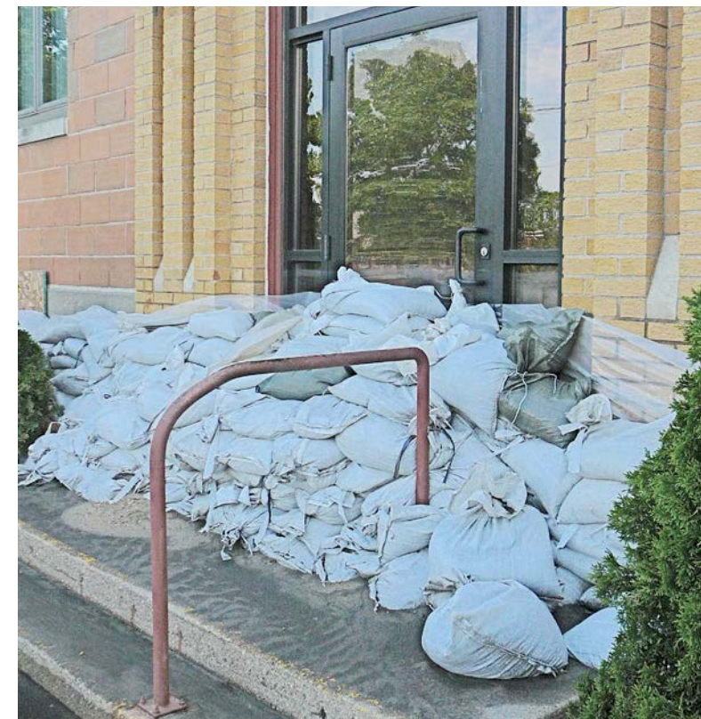
A wall of sandbags were piled against the parish house doors during the rising waters of the 2008 Cedar River flood.
