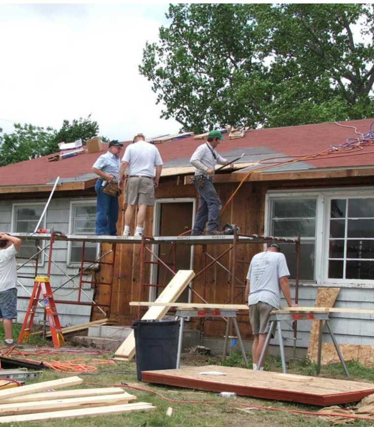
St. Paul's members volunteered on a Habitat construction project.
