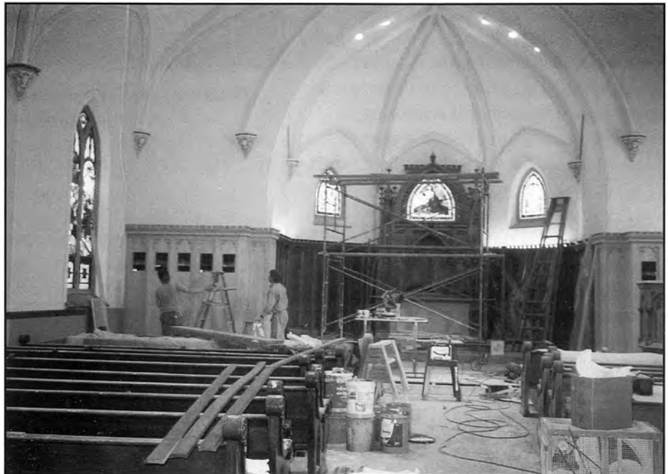
Work on the sanctuary refurbishing was under way in 1992
