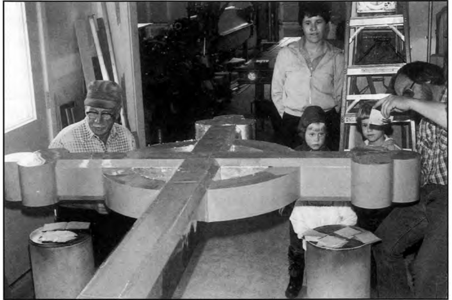
Dave and Alan Hamilton worked with thin sheets of gold leaf as they regilded St. Paul's steeple cross
