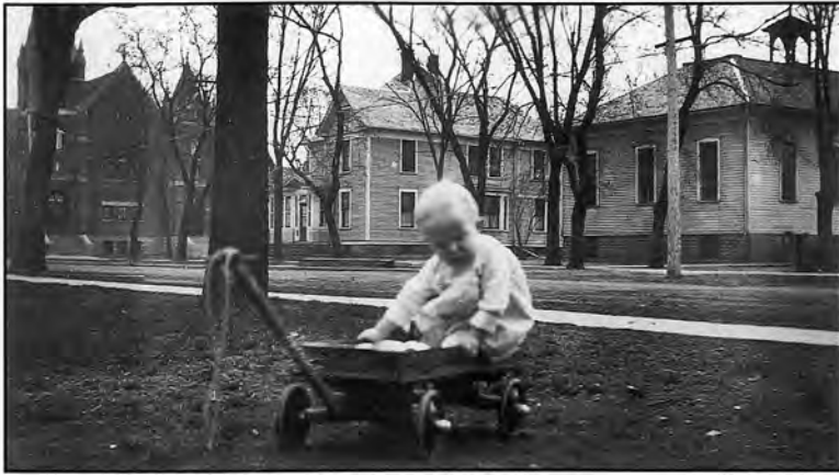
St. Paul's School building erected in 1890 near present school (Bldg. located on Hwy. 218 South)
